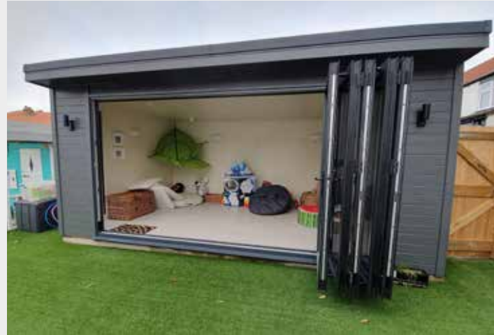
16' X 10' Pent garden studio, thermowood cladding, Aluminium 5 leaf 12ft bifold doors, painted finish in charcoal, MDF (V grooved) painted lining (white) with breathable membrane (moisture barrier) and Celotex insulation, painted finish in charcoal, EPDM rubber roof, laminate installed by customer & black guttering
